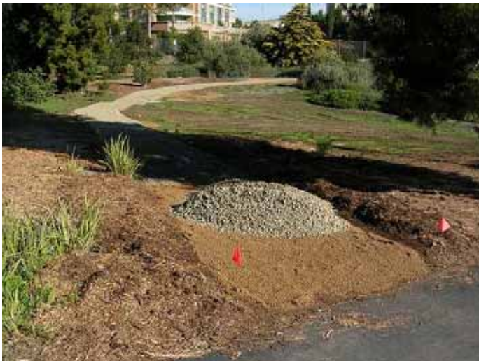
Progress Photo of New Path in California Gardens
